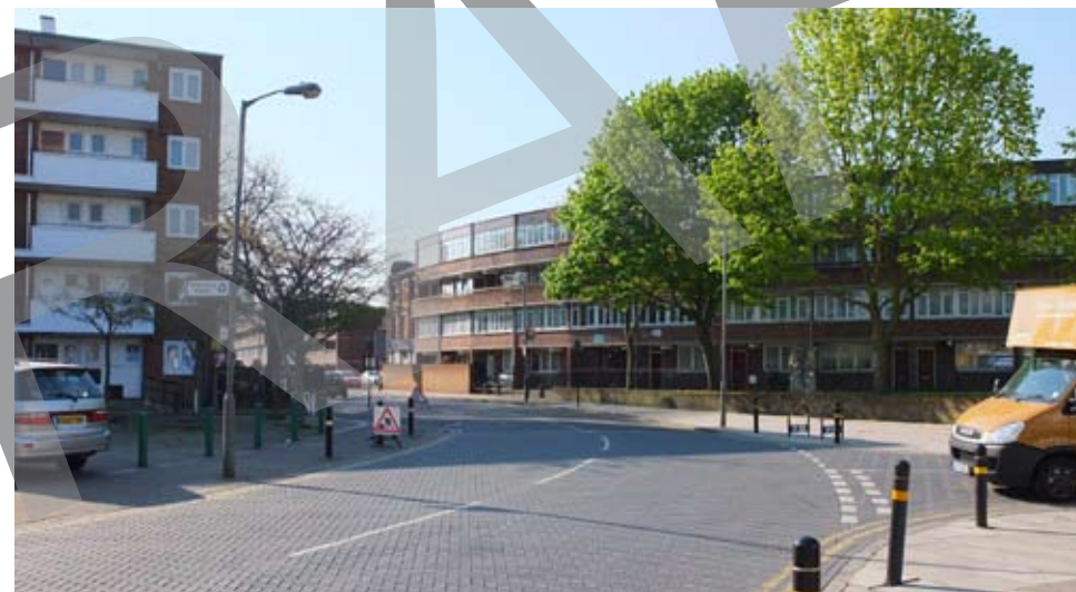
Raised tables reduce traffic speeds at junctions and can use attractive materials
