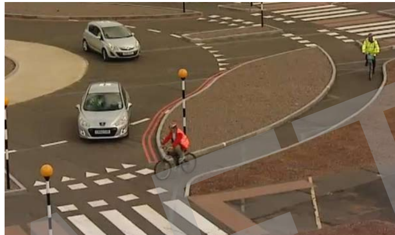
Cycle tracks segregated through roundabouts (undergoing trials)
